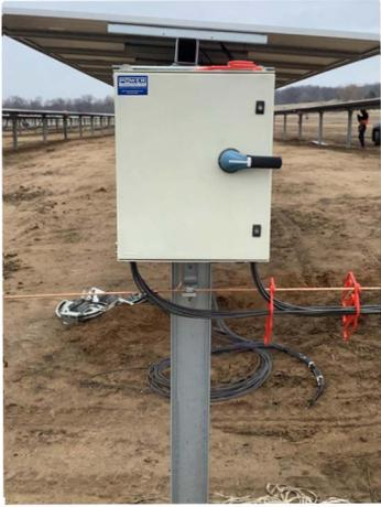
Secure the enclosure to the struts at all four tabs, using appropriate 5/16-inch fasteners, washers and nuts (not supplied)
