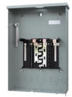
SIEMENS LOW VOLTAGE PLUG-ON NEUTRAL READY STANDARD SERIES ASSEMBLED LOAD CENTER. MAIN LUG WITH 12 1-INCH SPACES ALLOWING MAX 24 CIRCUITS. 1-PHASE 3-WIRE SYSTEM RATED 120/240V (200A) 100KAIC. SPECIAL FEATURES: ALUMINUM BUS, GREY TRIM NEMA TYPE 3R ENCLOSURE FOR OUTDOOR USE.
